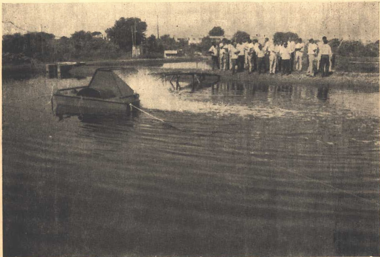
A view showing floating aerator in action in the pilot plant aerated lagoon.
