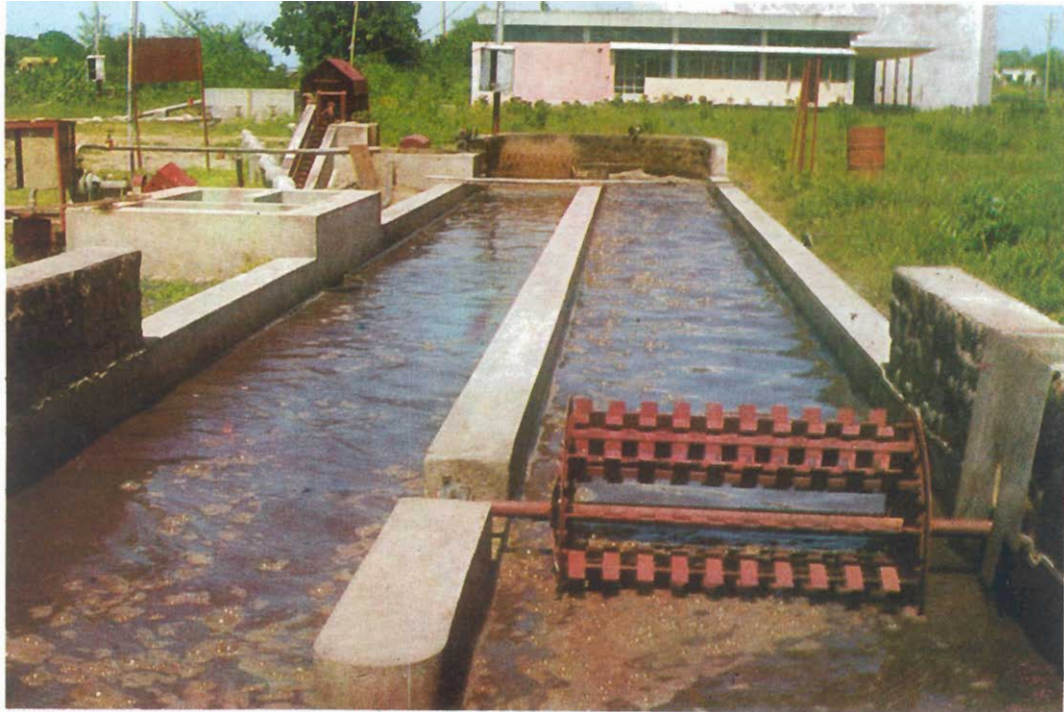
PASVEER TYPE OXIDATION DITCH
