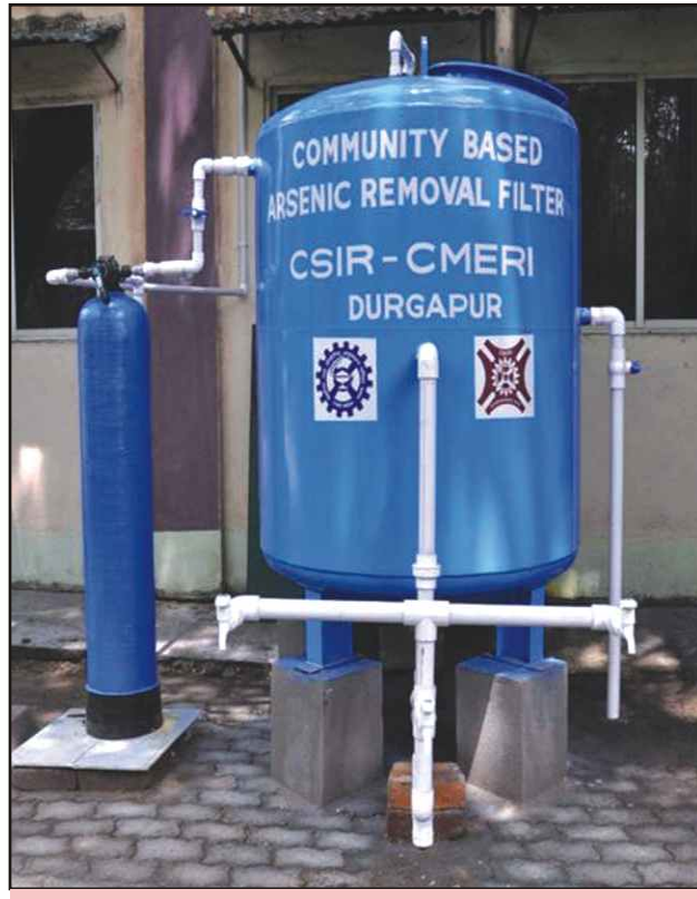
Community Level Arsenic Removal Filter-Model II at CSIR-CMERI
