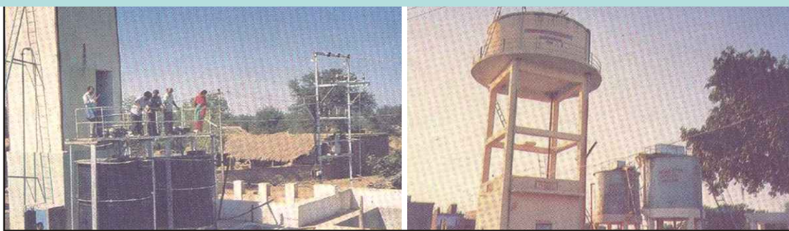
Fill-and-draw Defluoridation Plant at Badarpur, Gujarat
